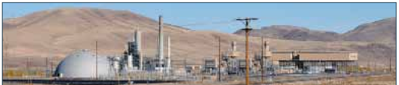
More than 900 megawatts of electrical power available directly to all park users.
